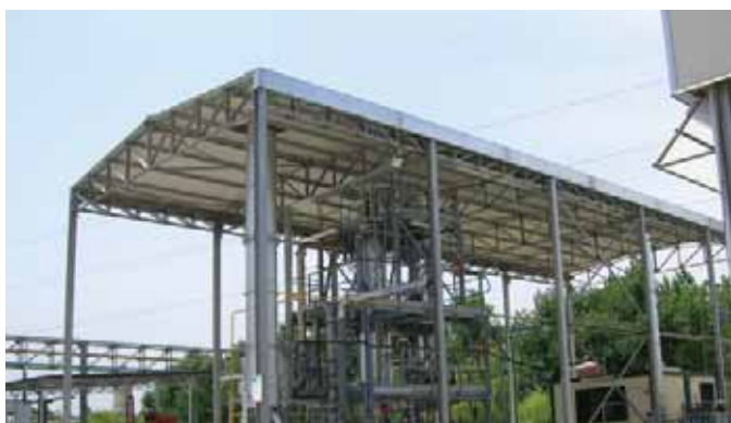
Fig. 2: AMRA FluGas Pilot Plant
